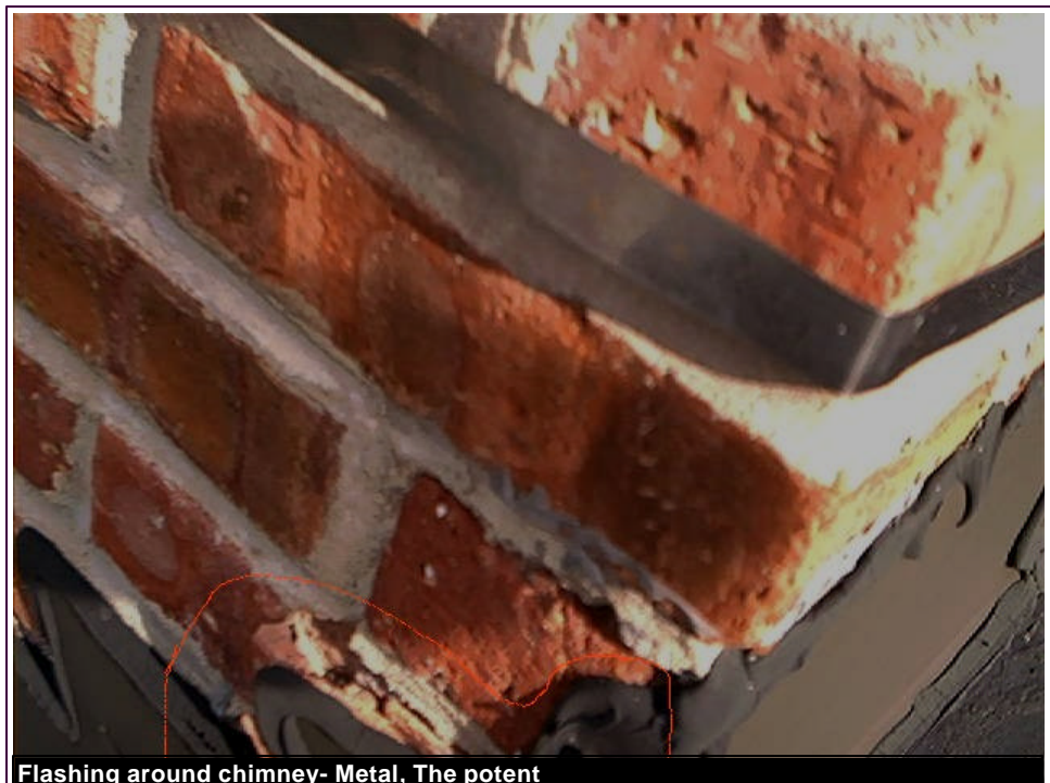
Flashing around chimney- Metal, The potent
